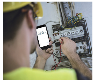
Electric Power Inspection
